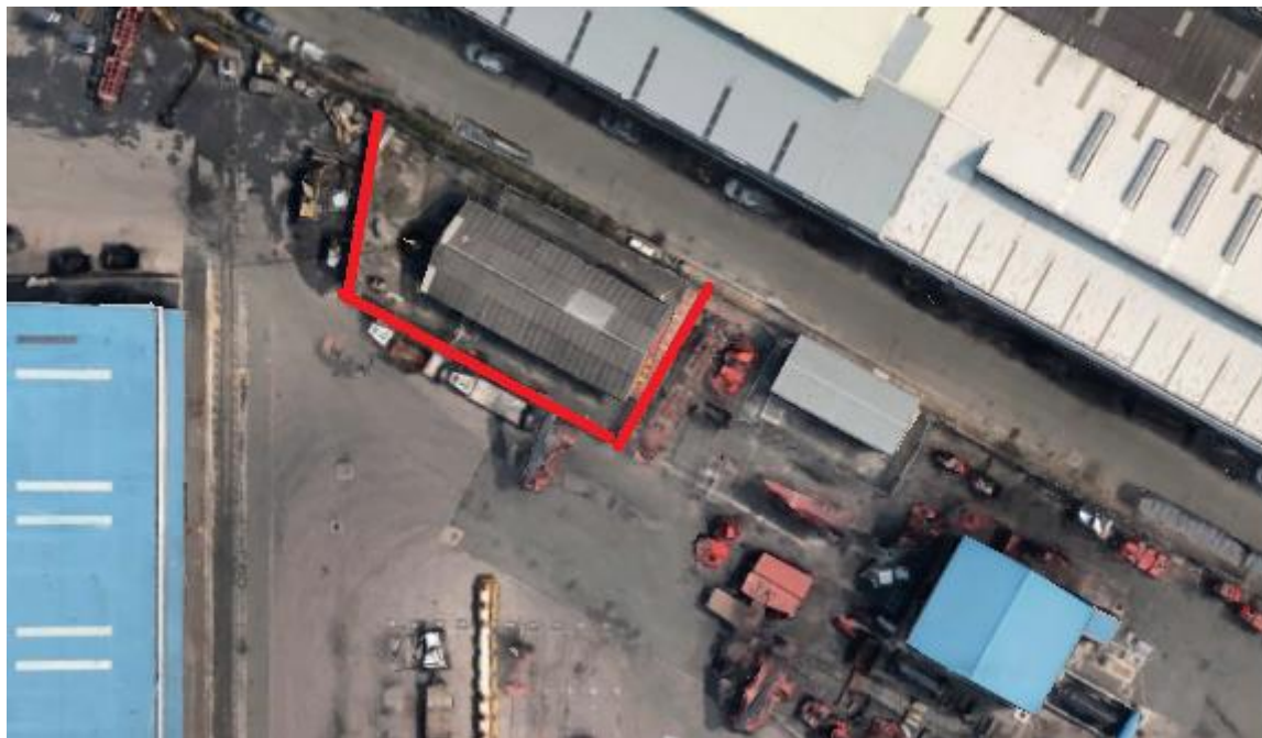
Figure 11: Maydon Shed 12 M & A
