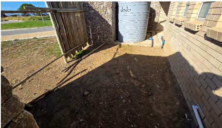
POLE SCREENS TO YARDS NOT SECURED & INCOMPLETE ON RIGHT SIDE YARD PAVING & GATES NOT DONE
