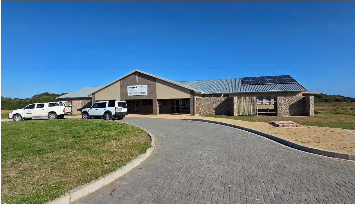
DAMAGED BARGEBOARD ON RIGHT SIDE & ALL EAVES & BARGEBOARDS TO BE REPAINTED WEEDS IN PAVING
