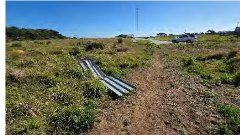
RUBBLE & OLD MATERIALS NOT REMOVED
