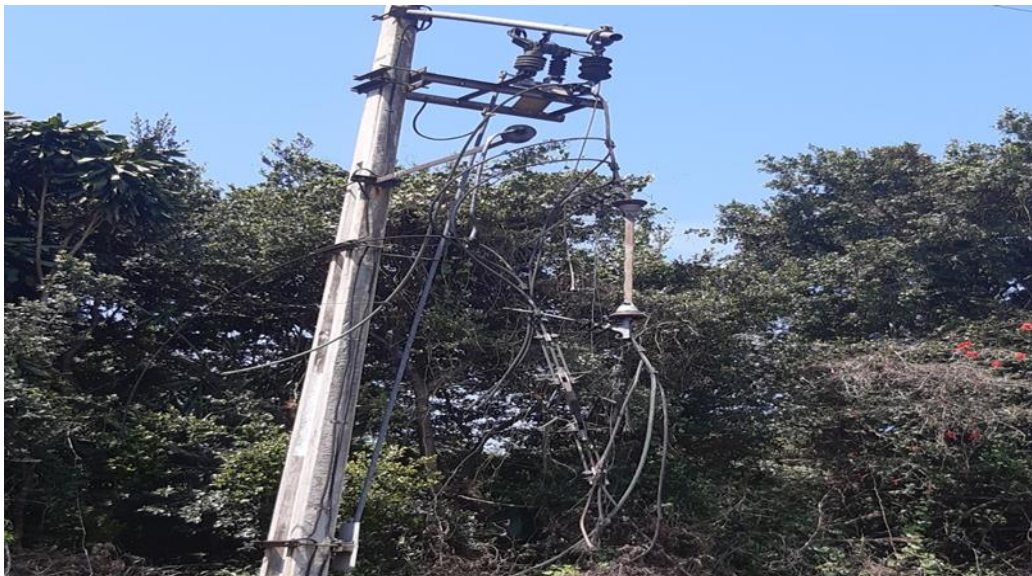
Picture1 stolen wires and track switch vandalised
