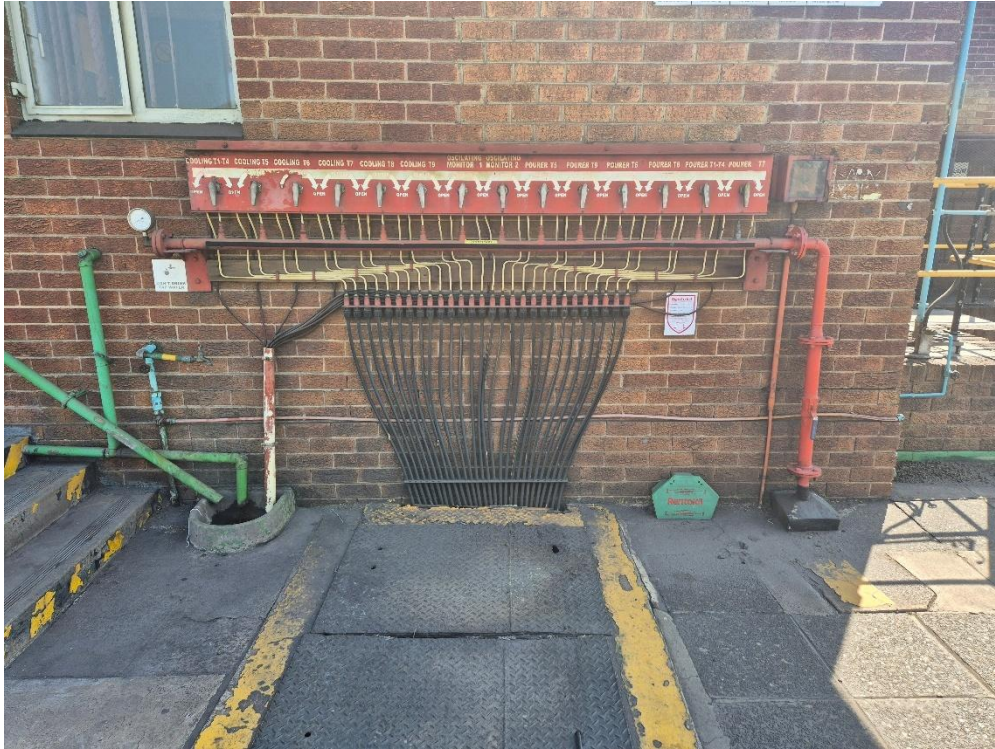
Figure 6: The figure above displays the existing remote hydraulic fire system activation manifold
