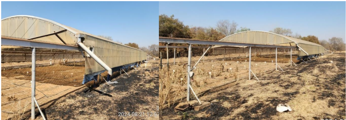
Photos of existing ARC structures
