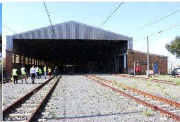
Figure 5: Current Shed West Entrance
