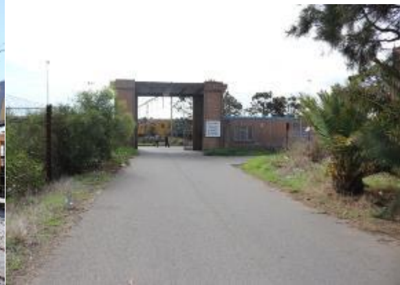
Figure 3: Entrance on Sunny Side Crescent
