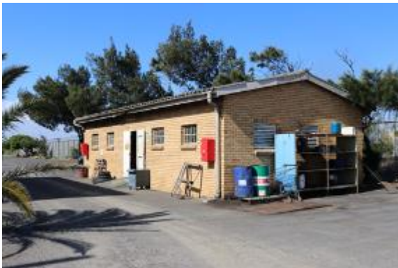
Figure 4: Oil Store Room
