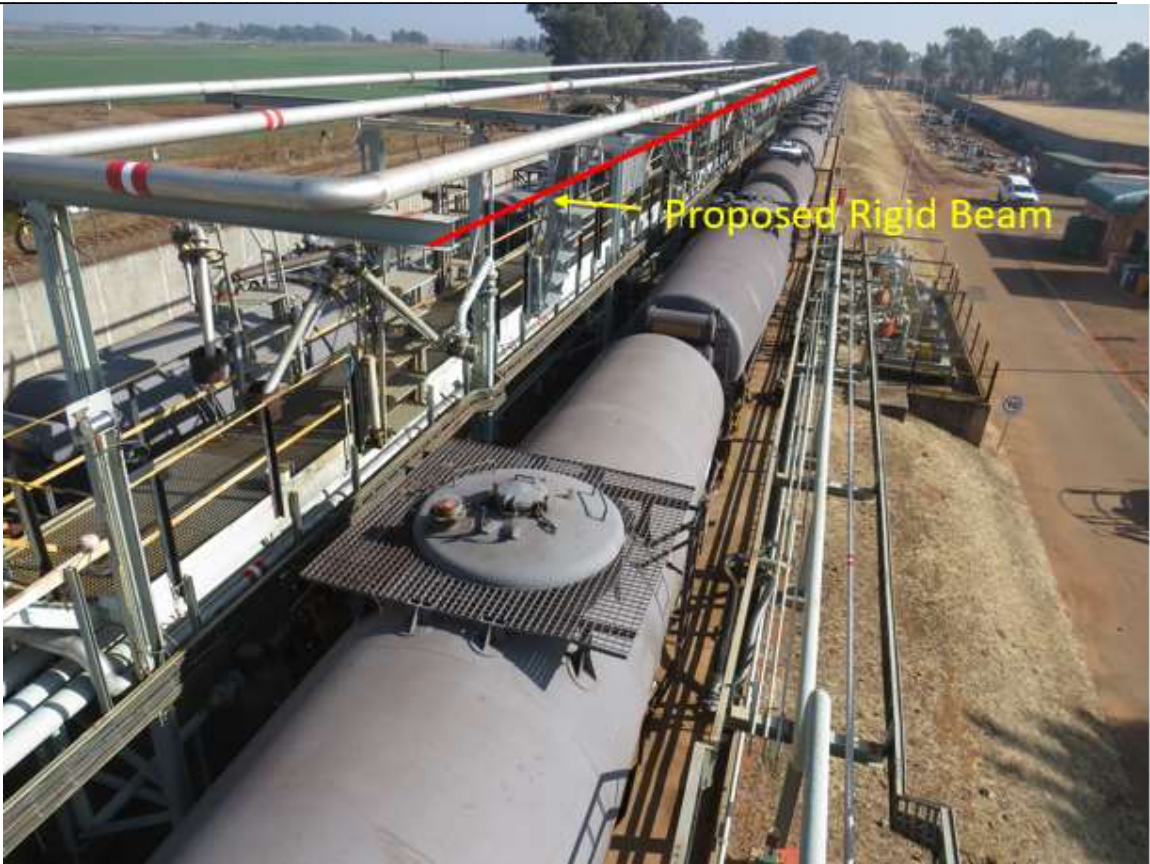
Figure 2: Current Rail Tanker Loading Facility at Tarlton Depot indicating the proposed Rigid Rail Fall Protection System Solution for Road Loading Facility
