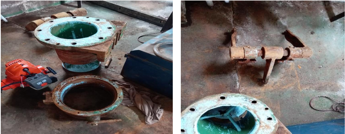
Figure 1: Redundant Sleeve valve and valve hood and stroke bracket
