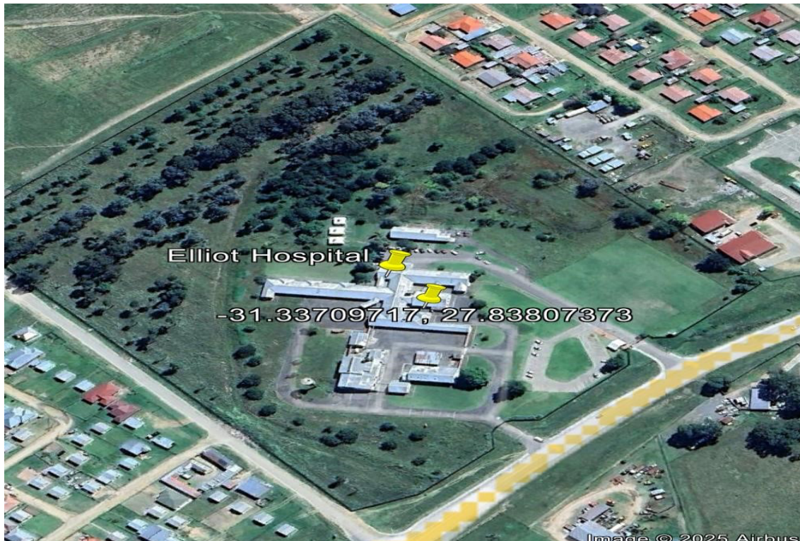
ELLIOT HOSPITAL AERIAL VIEW (SOURCE GOOGLE EARTH)
