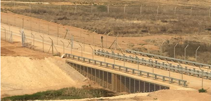
Figure 7: Security Grid Arrangement (Culvert/Bridge Crossing)
