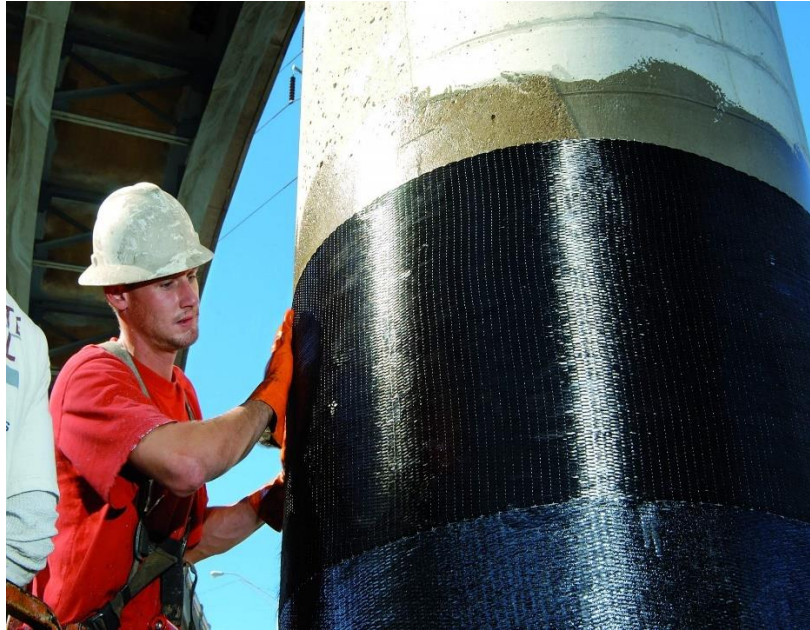
Figure 2: Sika Wrap Application
