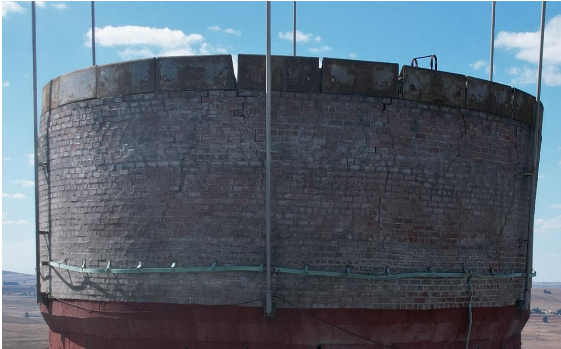
Diagonal brick wall cracks: Southern Chimney
