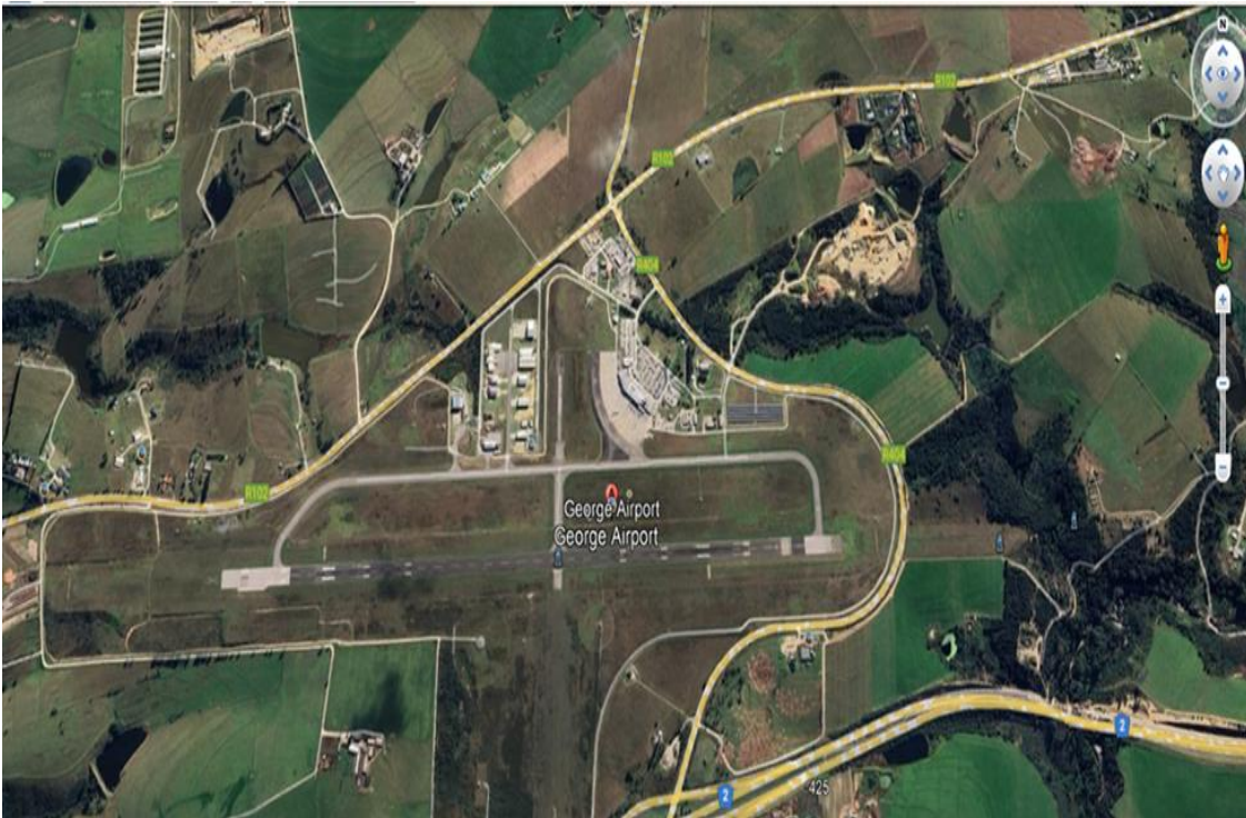
Figure C4.1: GRJ Aerial View Image
