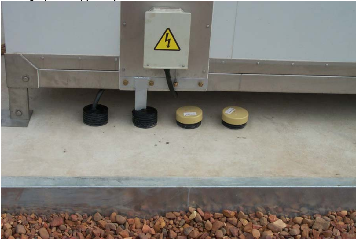
Photograph 1 Copper T-piece connection.
