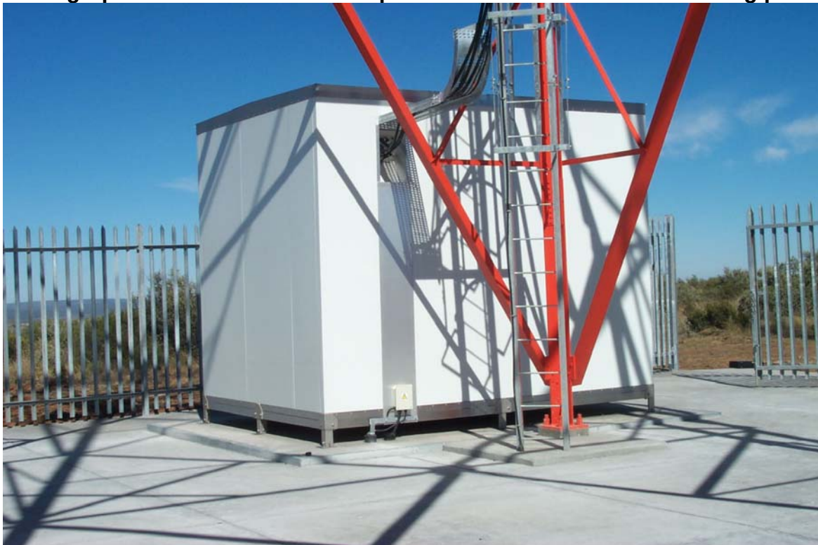
Photograph 2 Broad aluminium strip is used to bond RF & AC earthing points.
