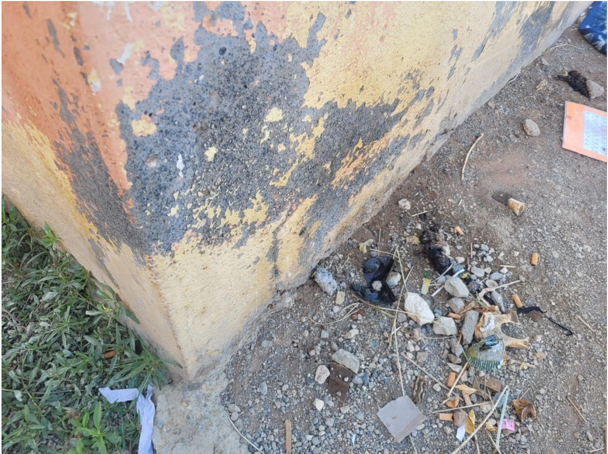
The foundation is a strip foundation no movement or settlement evident.
