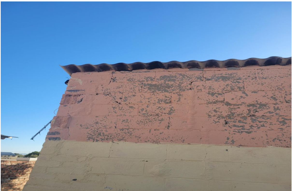
Longitudinal cracks due to no brickforce evident and poor workmanship.
