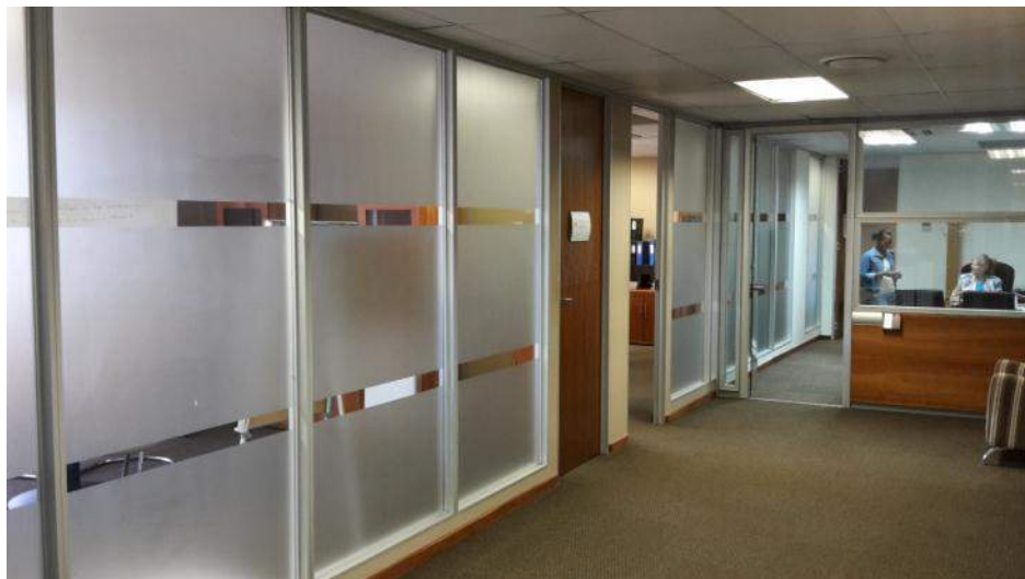
Figure 3-9 Full-height, modular frosted glazing panels with anodized aluminium frames
