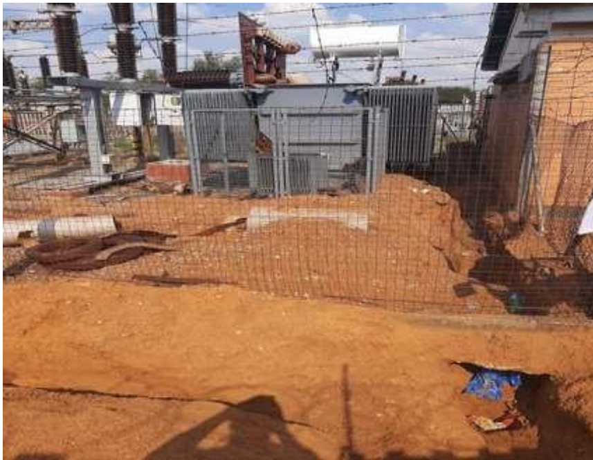
Figure 2.1: 88kV AC Outdoor Vandalised Equipment
