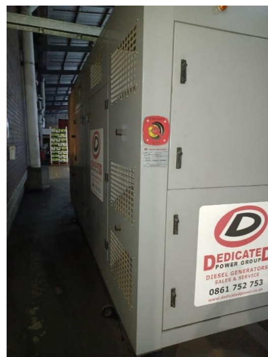
Figure 4: 11kV 220kVA Standby Generator
