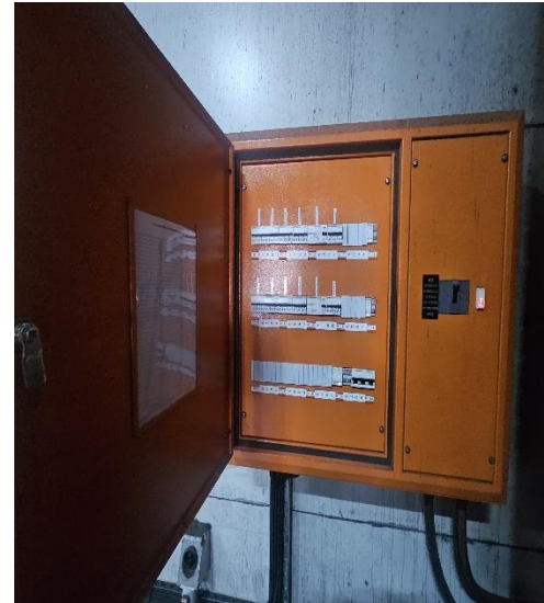
Figure 8: DB in good condition
