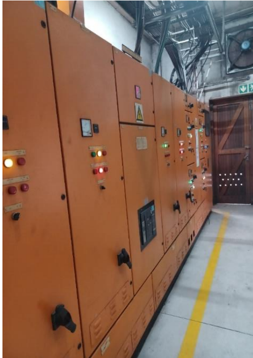
Figure 1: 11 kV and 400V switchgear
