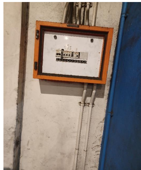
Figure 6: DB missing a door
