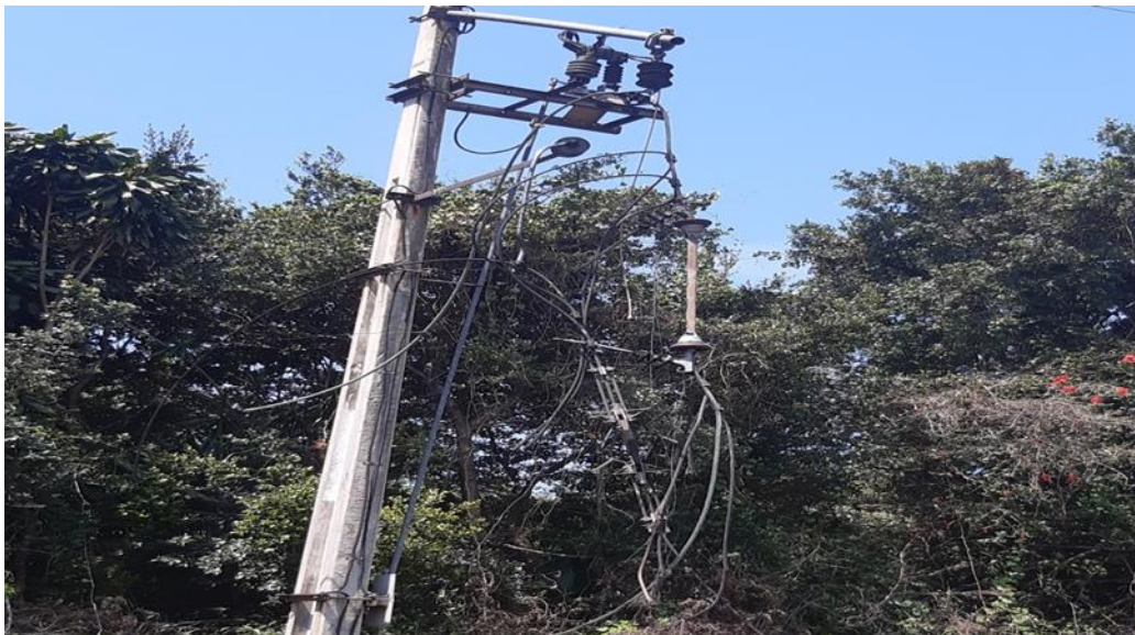
Picture1 stolen wires and track switch vandalised
