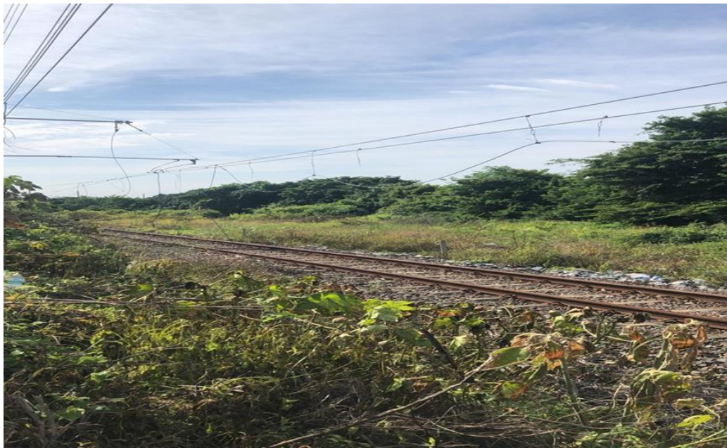
Picture 2 Contact wire and catenary wire hanging loose due to theft and vandalism
