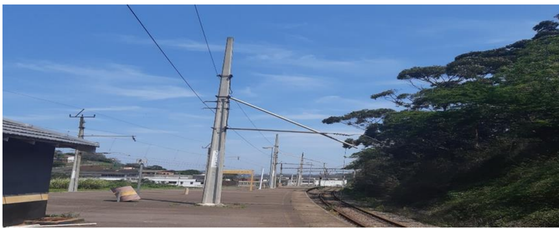
Picture 3: Stripped and broken tubular cantilever
