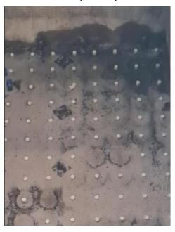
• The nozzles have a threaded end which screws into a threaded base which is imbedded into the sand filter floor. The threads on the embedded base are worn out and therefore the nozzles cannot be secured onto the sand filter floor. The Contractor is to repair/replace the sand filter embedded bases in order to ensure that the nozzles can be secured into the sand filter floor. The Contractor will also be required to inspect and replace any damaged nozzles.
