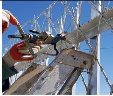
4. Stainless steel strapping for attaching diamond razor mesh
