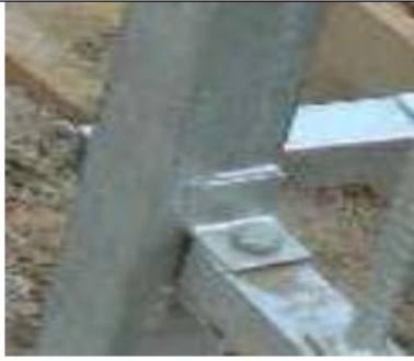
4. Palisade Post: L-shape tab with shear bolt and nut
