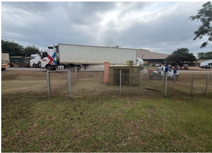
Start Point: Engine Garage Coordinates: -25.446329, 31.948437
