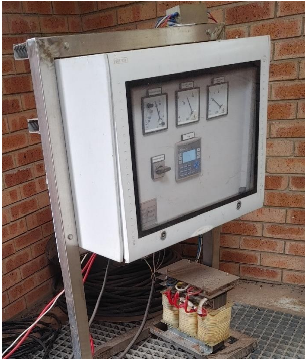
Fig, 1 – TRU with supply cables
