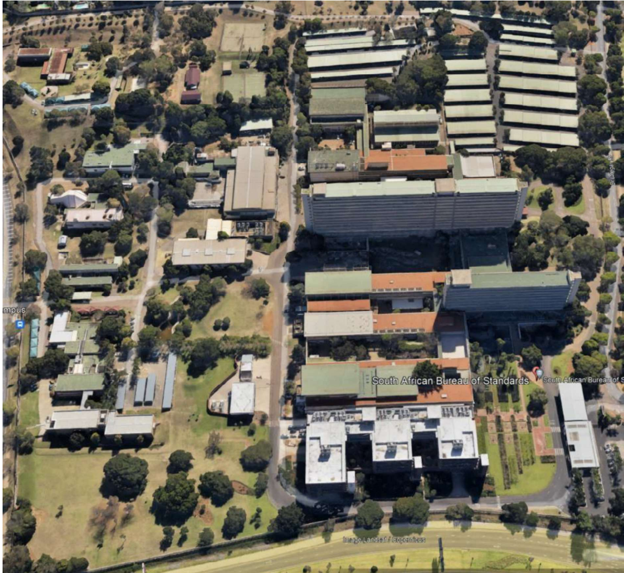
Figure 1. Aerial Site View
