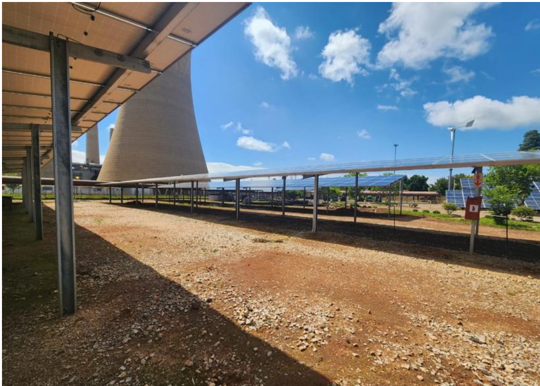
Figure 2: Existing PV plant where study is to take place.
