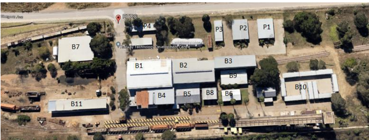
Aerial view of RTDC with the intended park-home installation area B10
