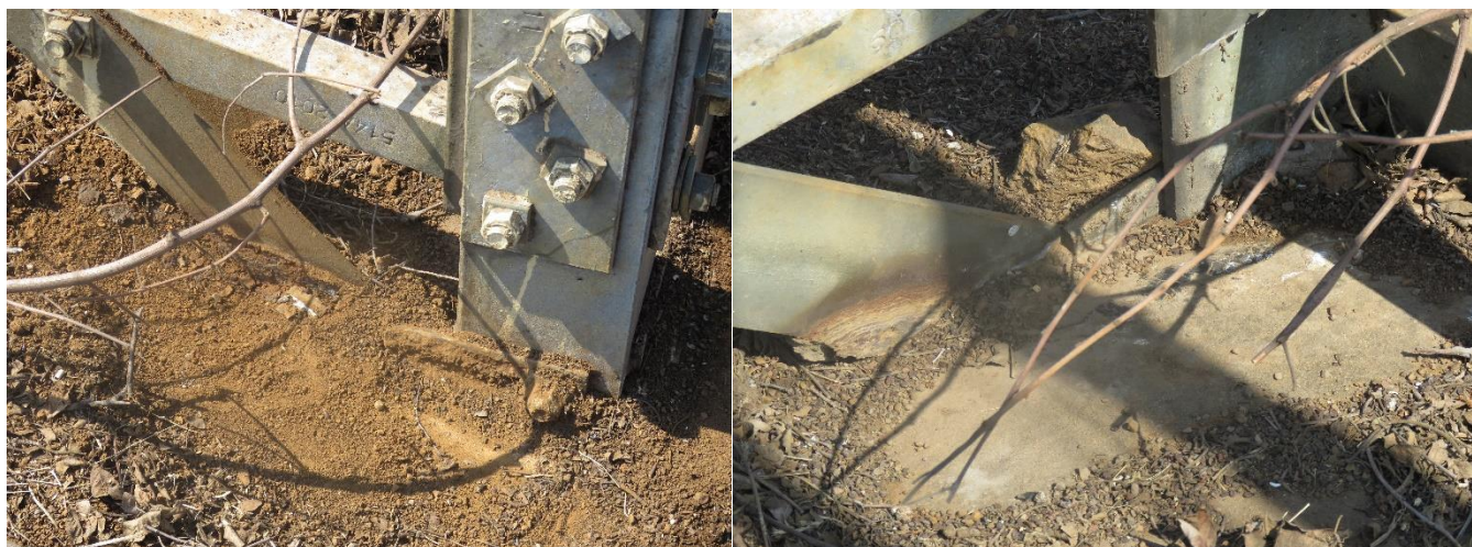
Figure 8: Corrosion on the stub and leg
