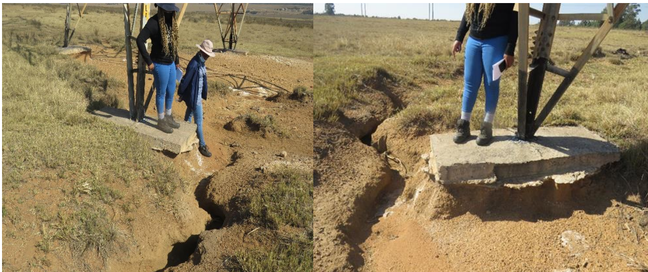
Figure 25: Scouring of foundations
