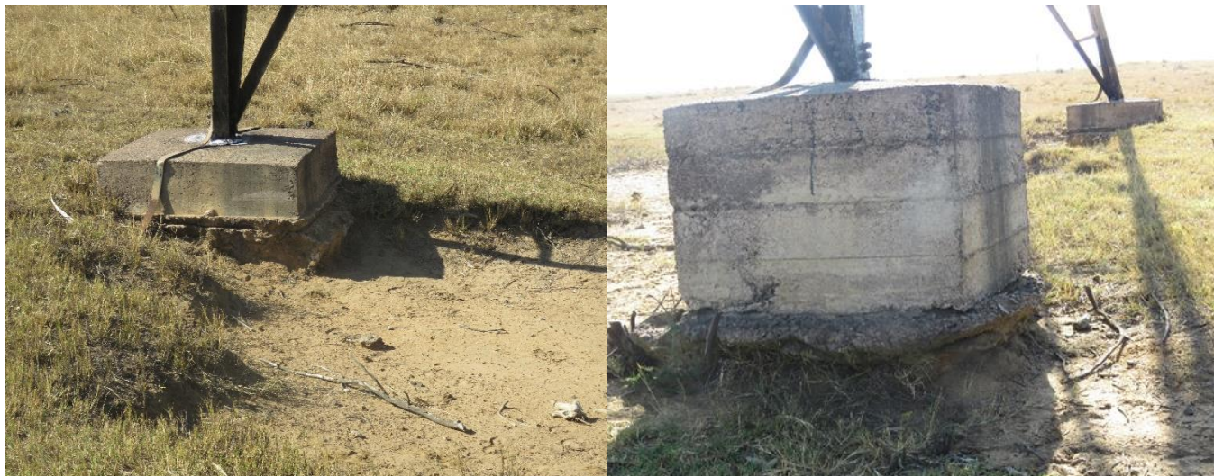
Figure 23: Scouring of foundation
