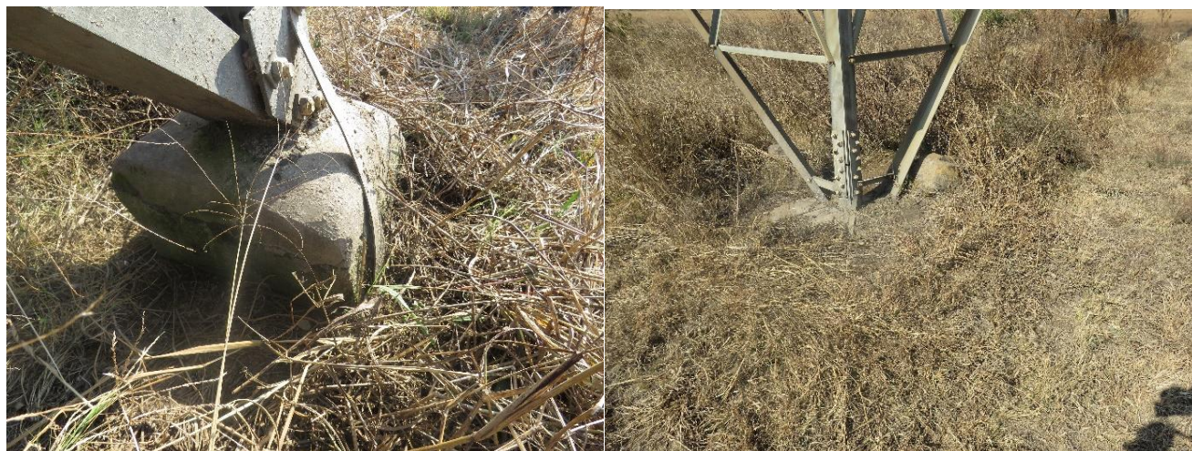
Figure 6: Concrete cracks and buried foundation
