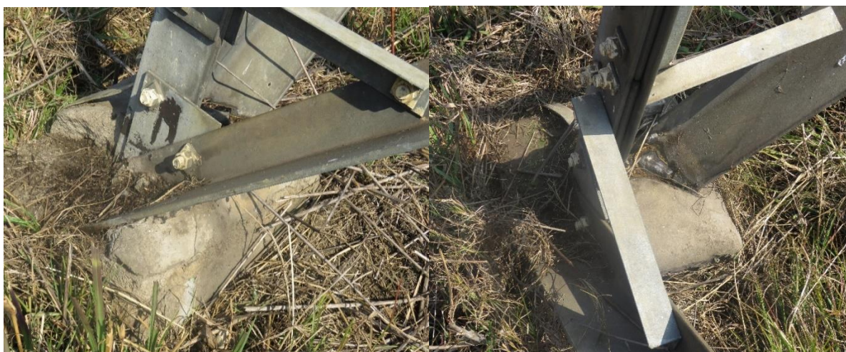
Figure 4: Cracked foundations
