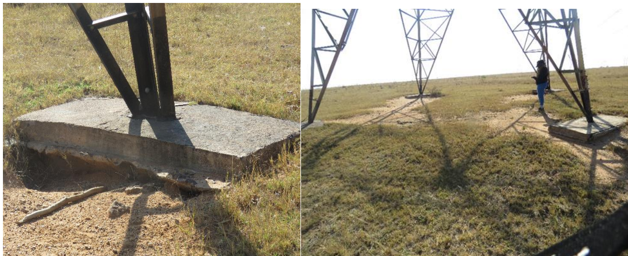
Figure 19: Scouring of foundation
