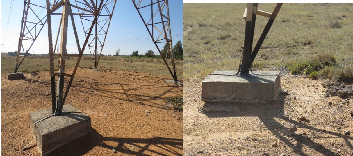
Figure 24: Scouring of foundations
