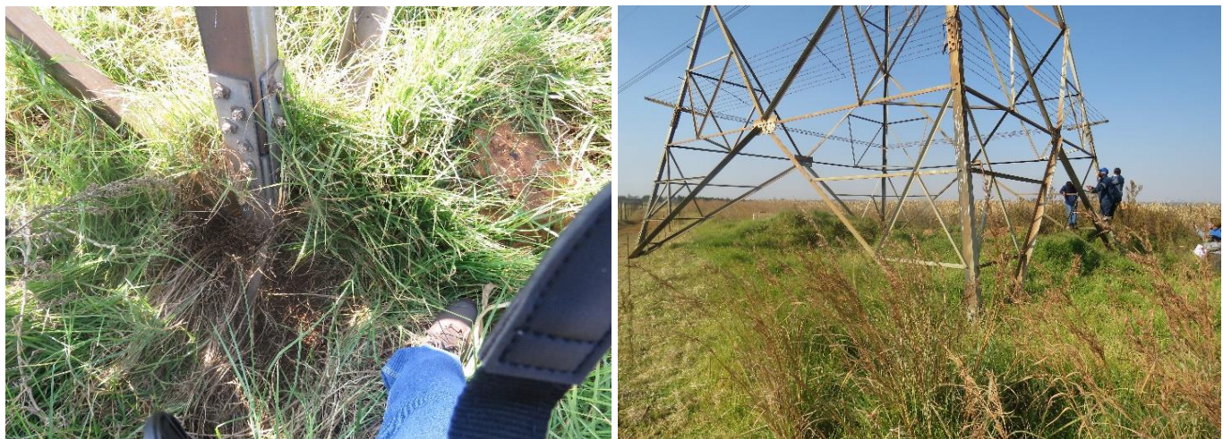
Figure 3: Foundations covered in vegetation
