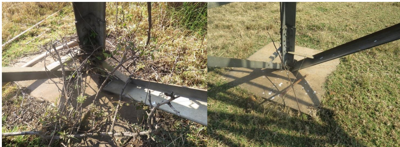
Figure 10: Buried foundations
