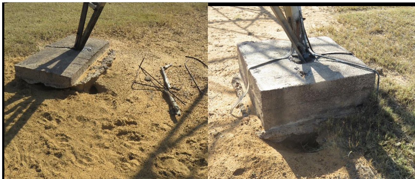
Figure 22: Scouring of foundation
