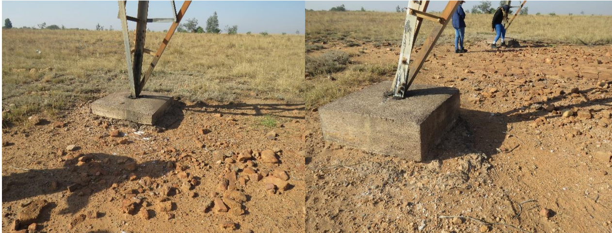
Figure 17: Scouring of foundations
