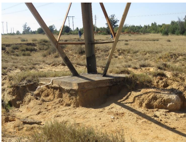
Figure 33: Scouring of foundation
