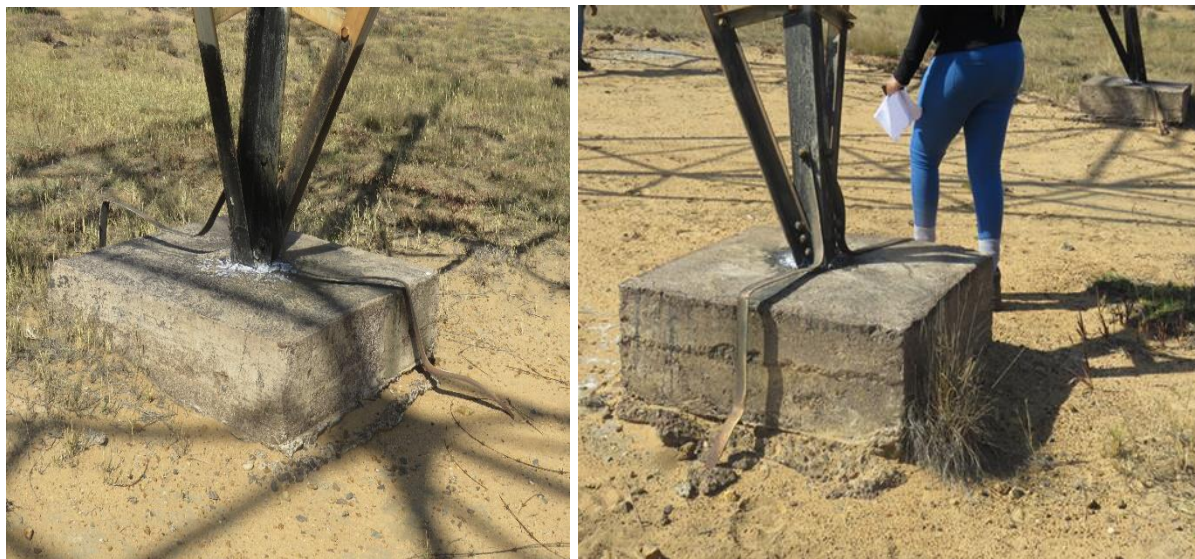
Figure 26 : Scouring of foundation
