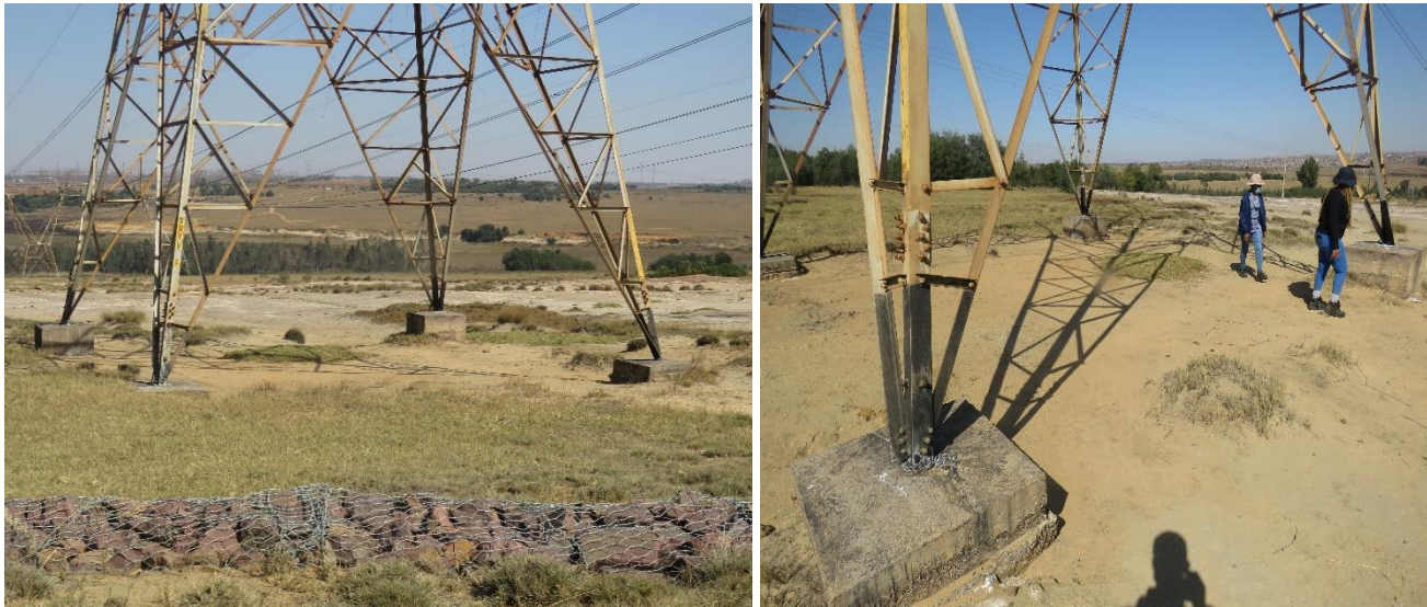
Figure 30: Scouring of foundations
