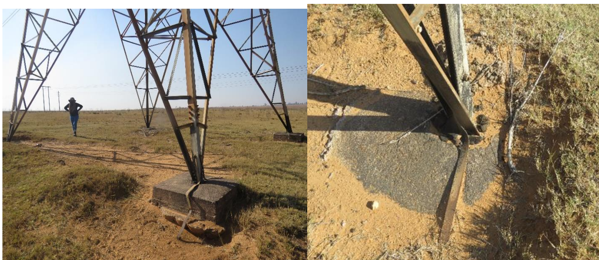
Figure 20: Scouring of foundation
