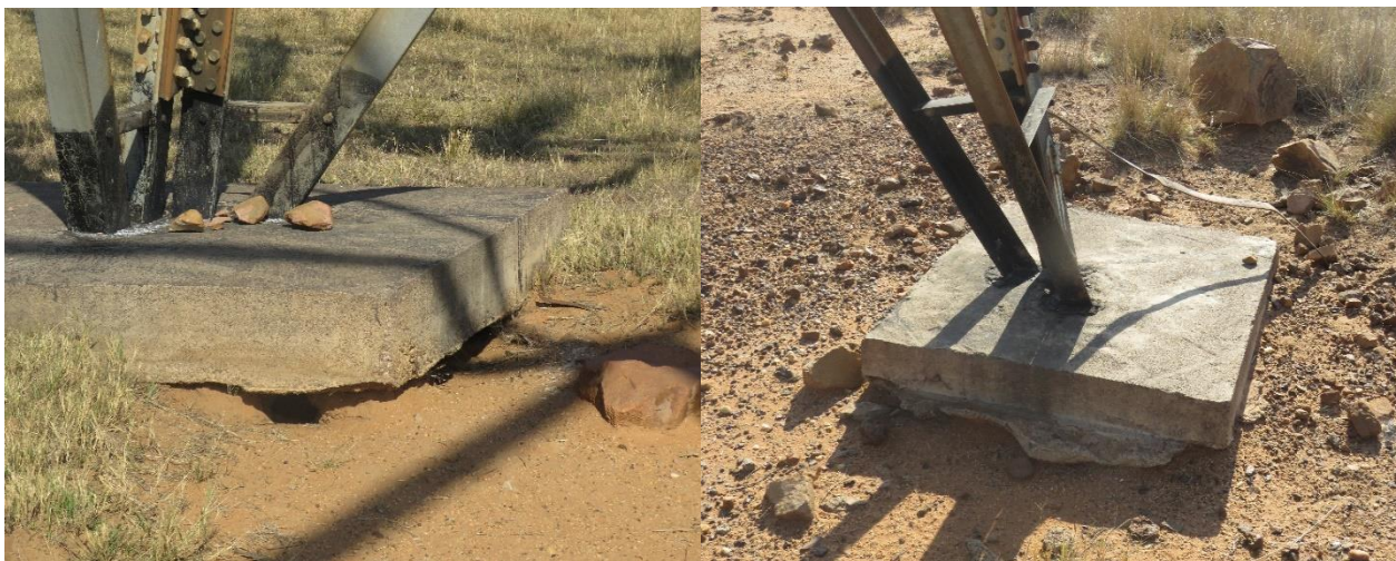
Figure 18: Scouring of foundation
