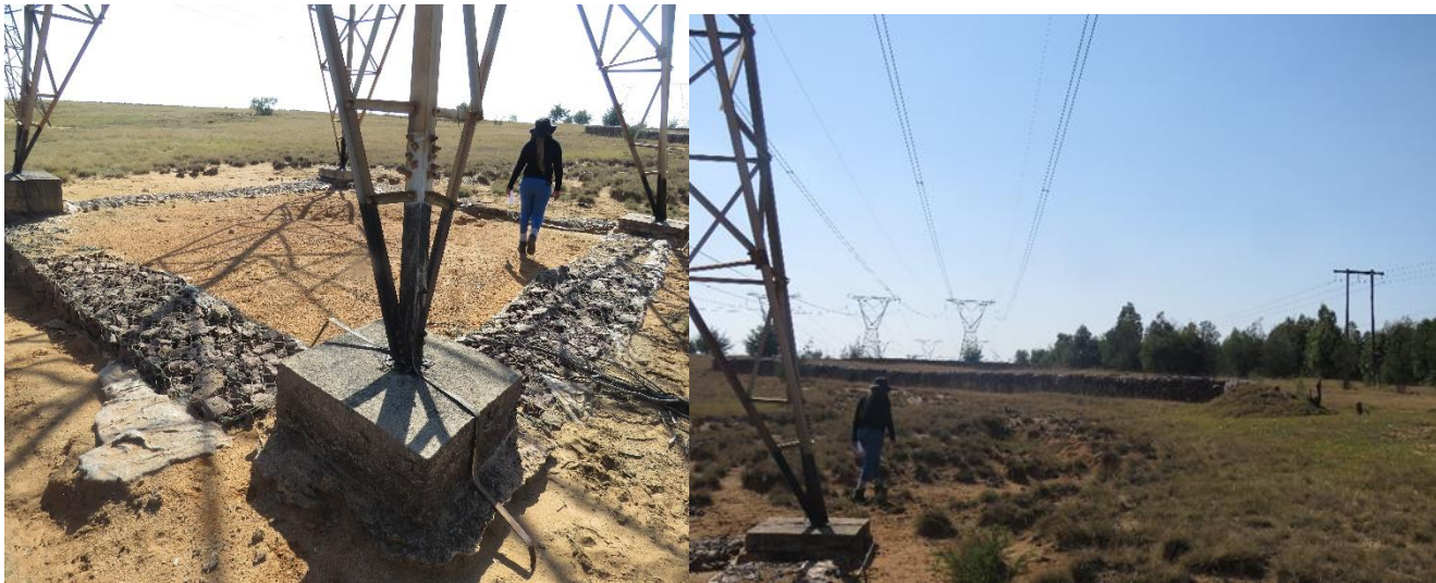
Figure 28: Existing Gabion Wall
