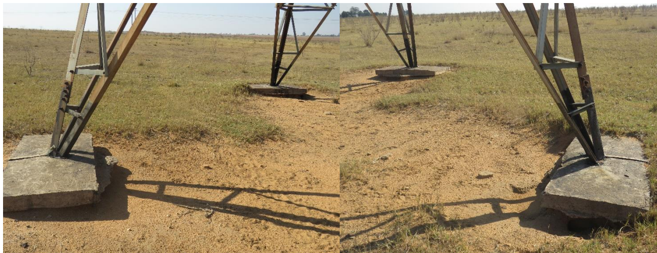
Figure 21: Scouring of foundation
