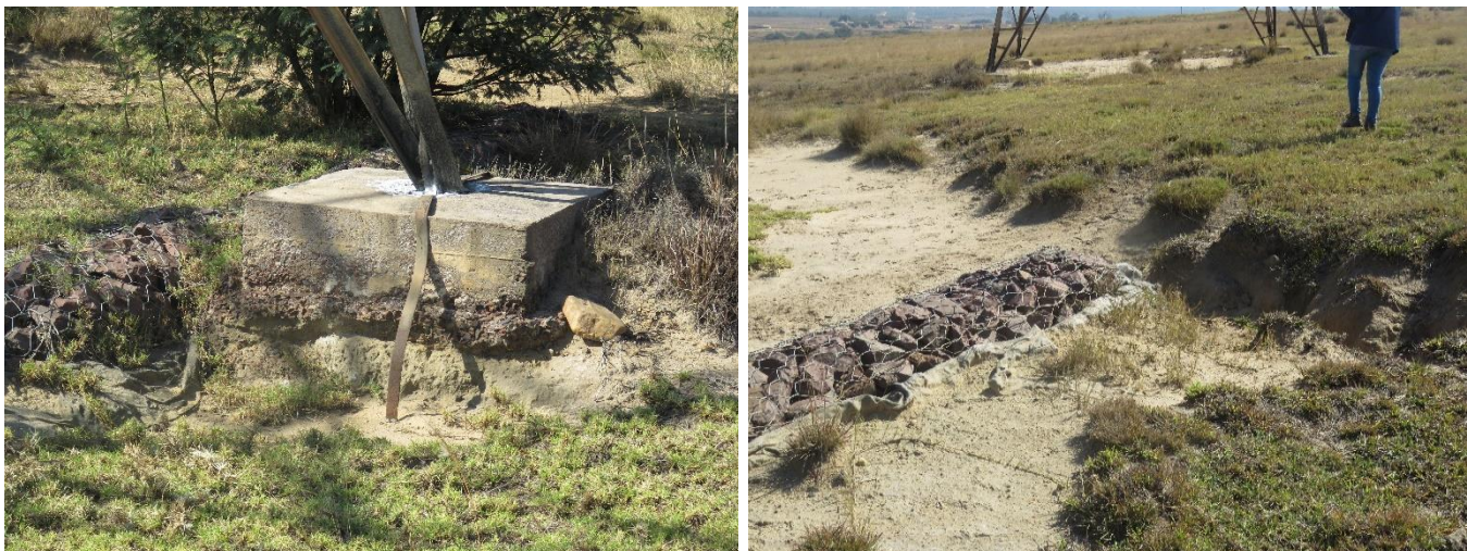
Figure 31: Scouring of foundations
