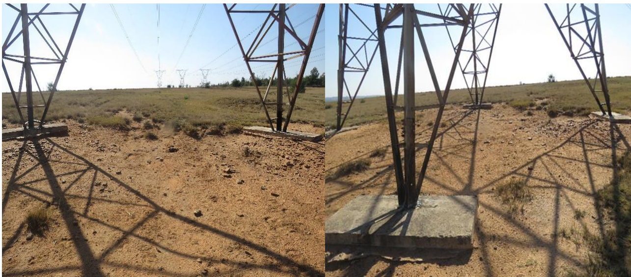
Figure 29: Scouring of foundations
