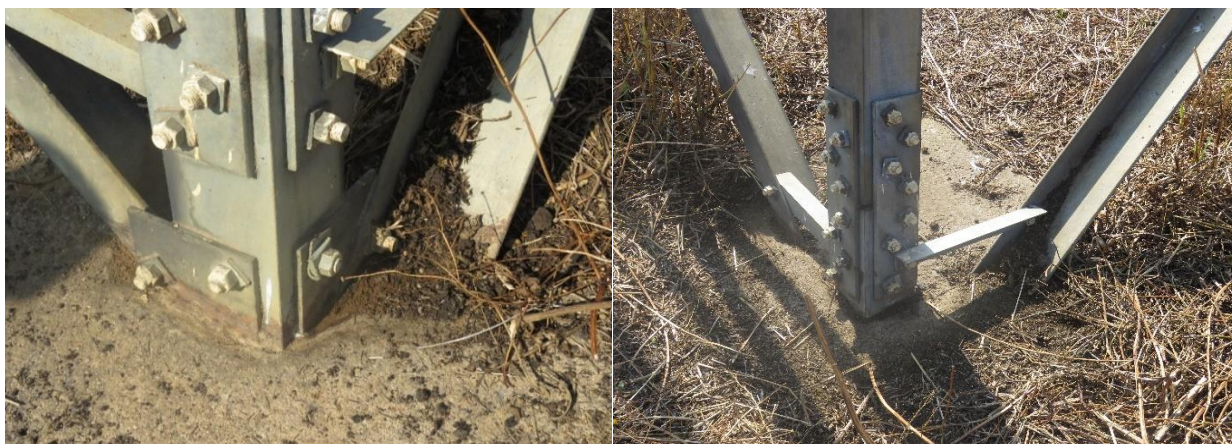
Figure 5: Corrosion on the stub
