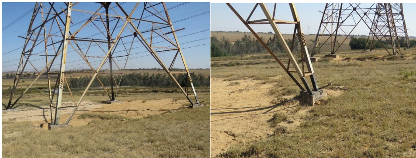
Figure 32: Scouring of foundations
