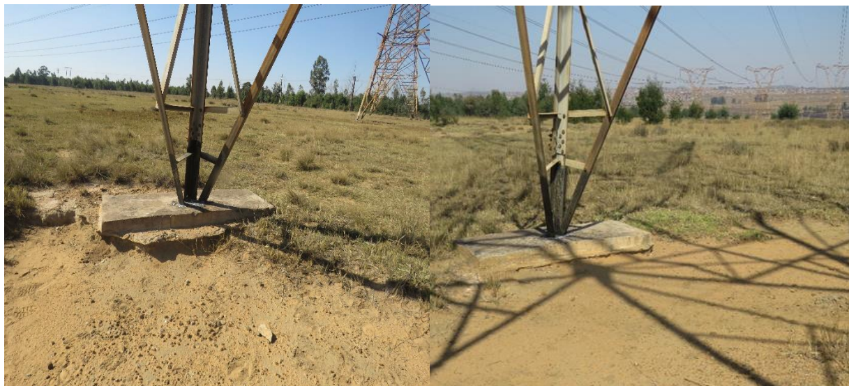
Figure 27 : Scouring of foundations
