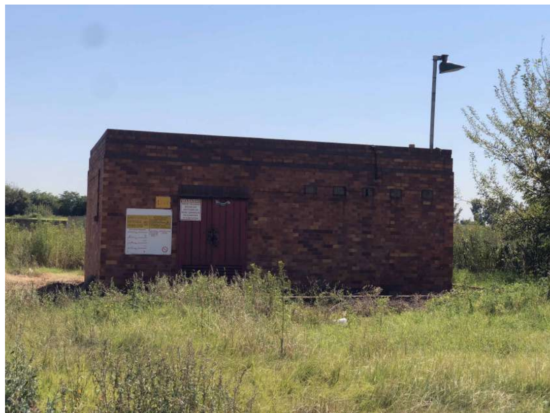
EXISTING SUBSTATION C
