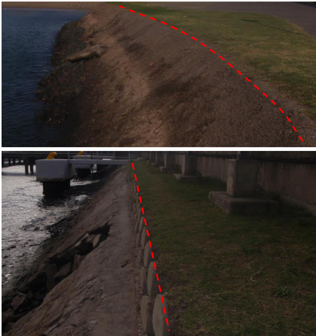
Figure 4-2: Examples of typical setting out lines.
