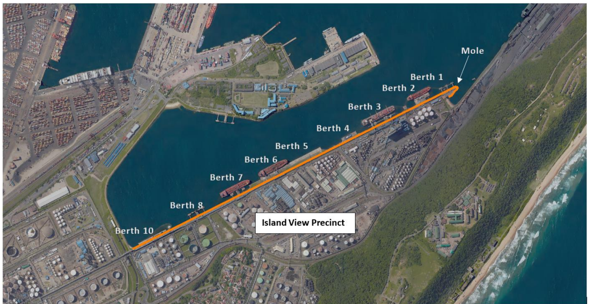
Figure 1-1: Island View Terminal
