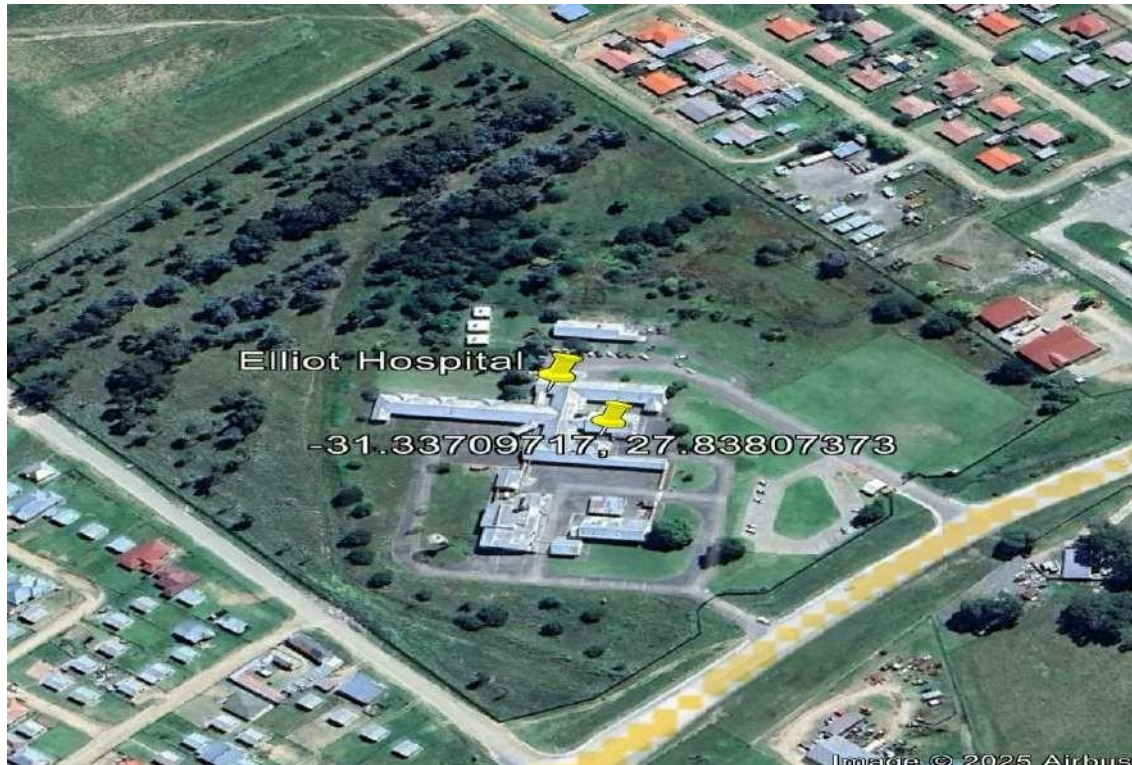
ELLIOT HOSPITAL AERIAL VIEW (SOURCE GOOGLE EARTH)
