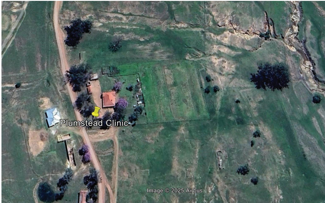
PLUMSTEAD CLINIC AERIAL VIEW (SOURCE GOOGLE EARTH)
