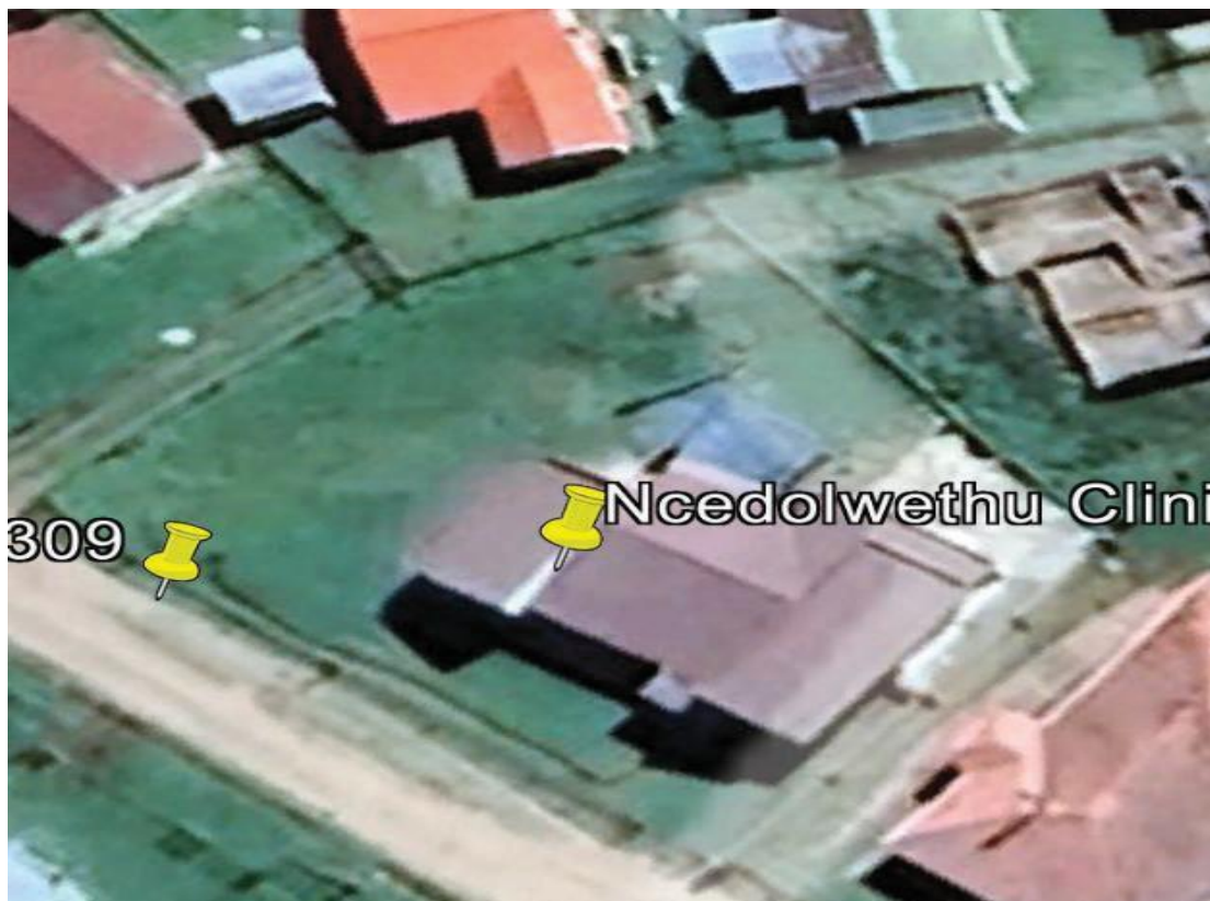
NCEDOLWETHU CLINIC AERIAL VIEW (SOURCE GOOGLE EARTH)
