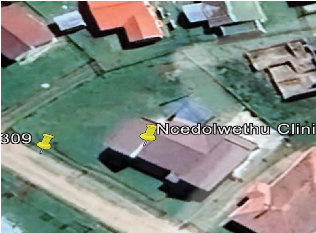
NCEDOLWETHU CLINIC AERIAL VIEW (SOURCE GOOGLE EARTH)
