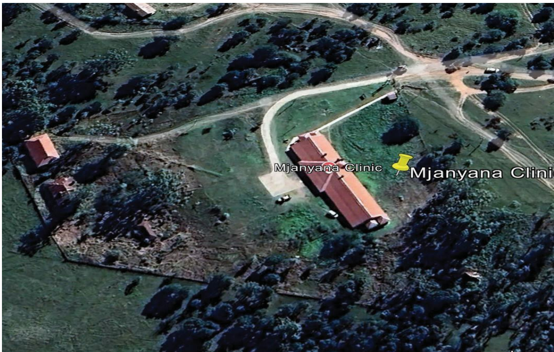
MJANYANA GATEWAY CLINIC AERIAL VIEW (SOURCE GOOGLE EARTH)
