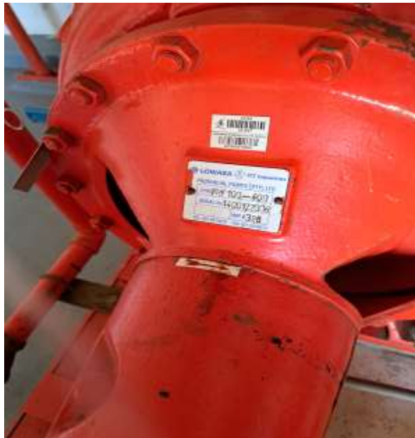
Fire Booster Centrifugal Pump Name Plate
