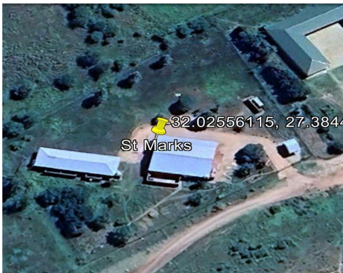
ST MARKS CLINIC AERIAL VIEW (SOURCE GOOGLE EARTH)
