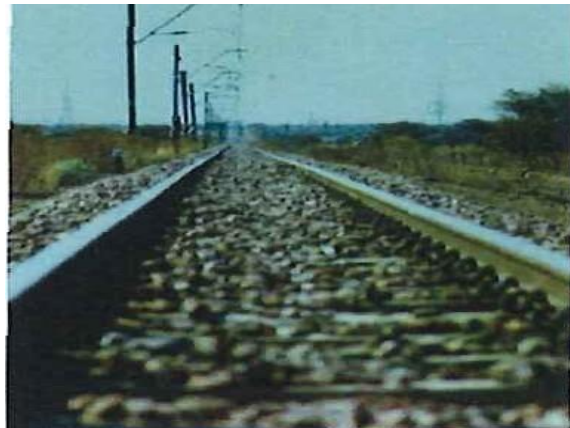
Figure 229: Tamping Removed the Defect to Restore the alignment
