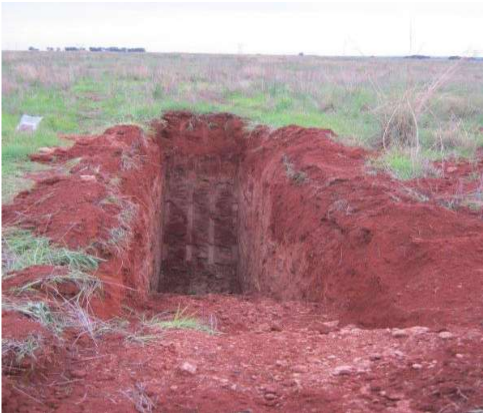
Photo 2: Test pit (TP) 12
