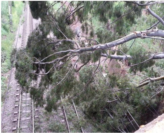
Figure 1: Trees falling on OHTE
