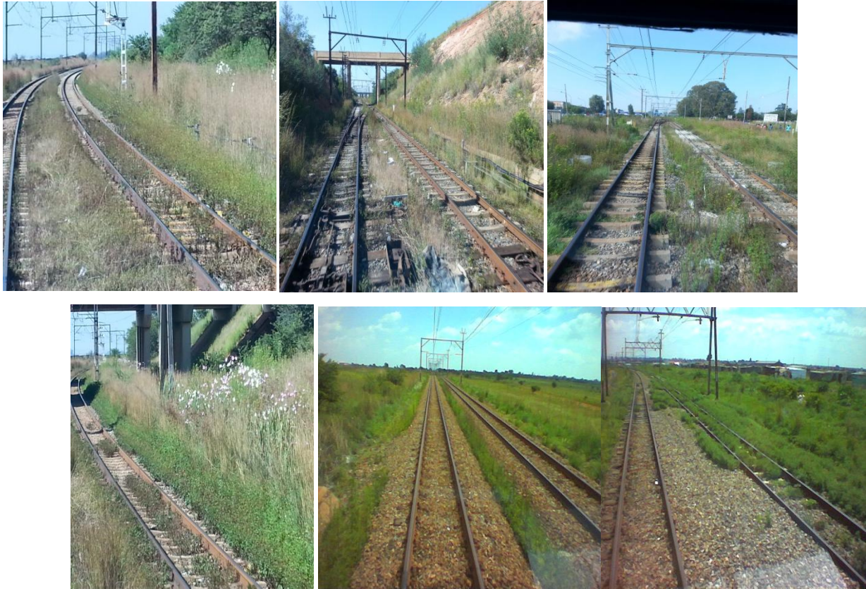
Figure 5: Overgrown vegetation on railway tracks.
