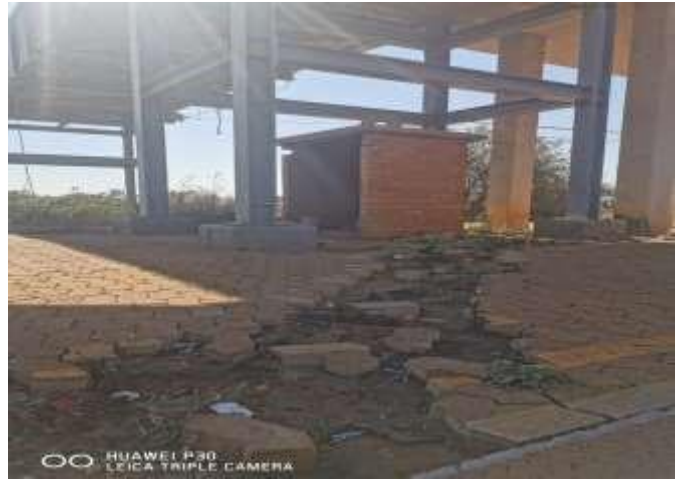
Picture 2: Damaged paving at the platforms
