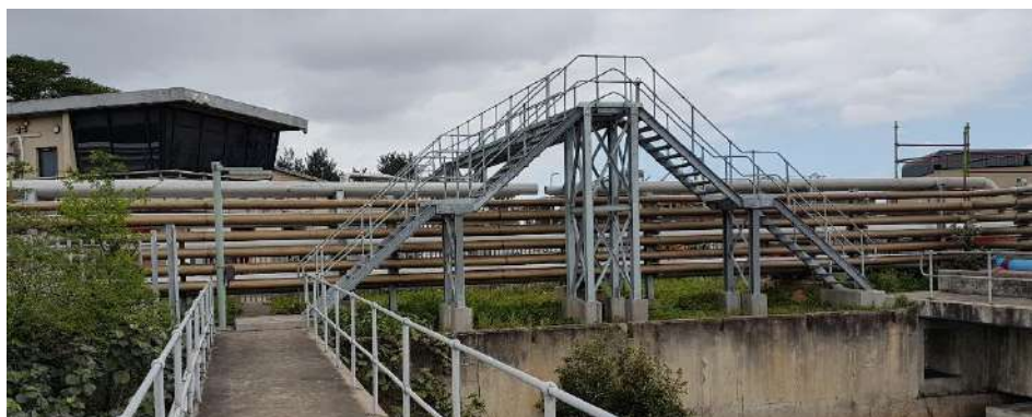
Figure 3-12: Access Walkway over Pipe Rack
