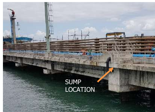
Figure 3-11: Stormwater Pump Sump
