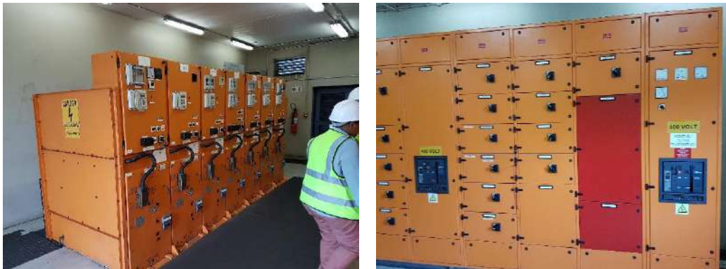
Figure 3-1: MCC & electrical panels in berth sub-station
