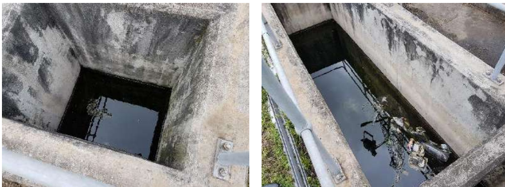
Figure 3-9: Water found within the Oil Trap
