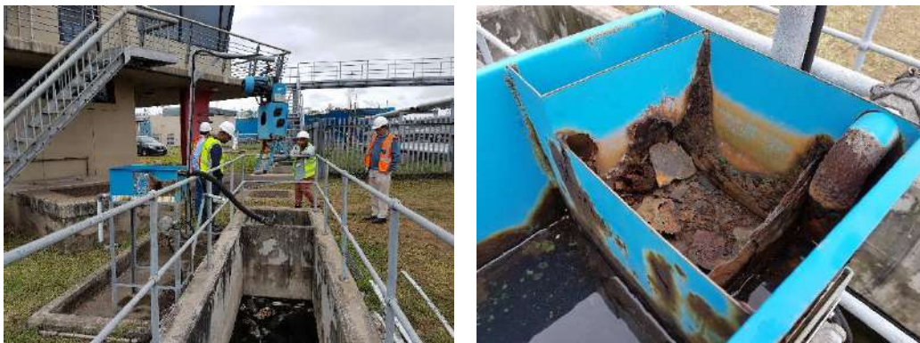
Figure 3-8: Oil Trap Sump and Collection/Skimming Mechanism
