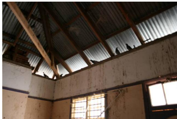
INTERNAL CEILINGS HAVE COLLAPSED FROM PIDGEON INVASION
