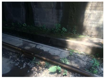
**Figure 4:** Broken track slab due to slab deformation and excessive settlement. Evident surface water resulting in unstable underlying track formation.
