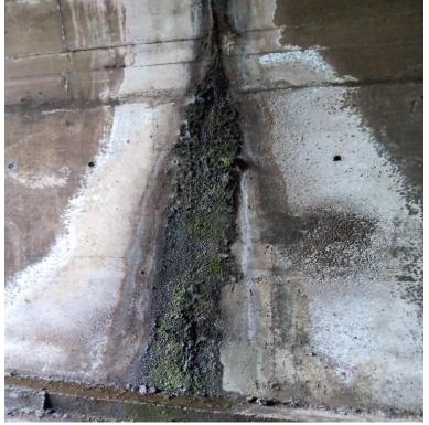
**Figure 5:** Cracking concrete walls of the portal due to water seepage from the top soil and enchroachment.
