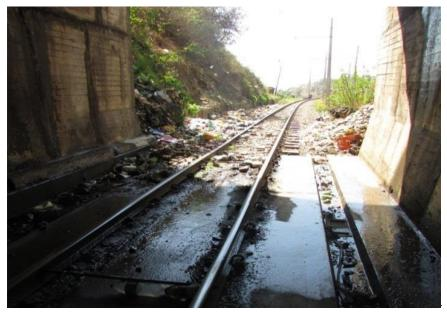
Figure 3: Poor drainage, fomation settlement and track widening at Zwelethu Tunnel
