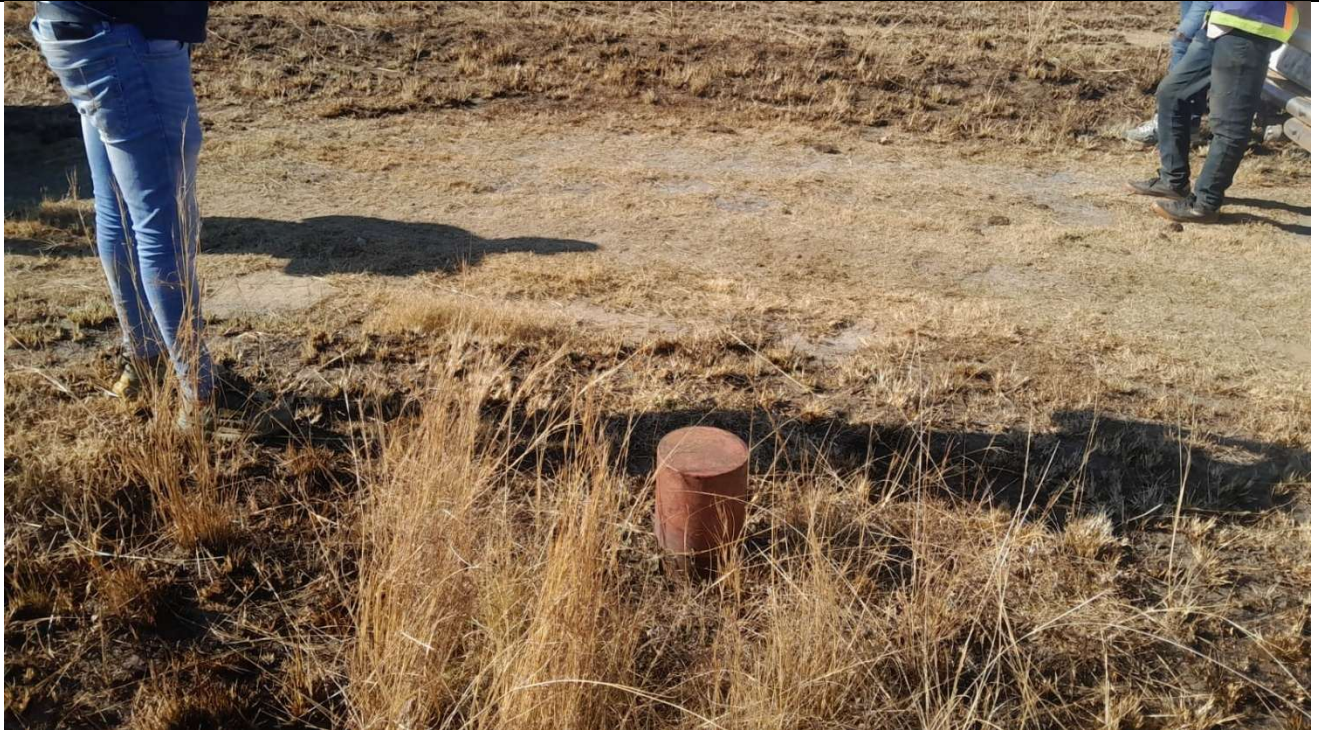
Photo 7: Existing Borehole (unequipped)
