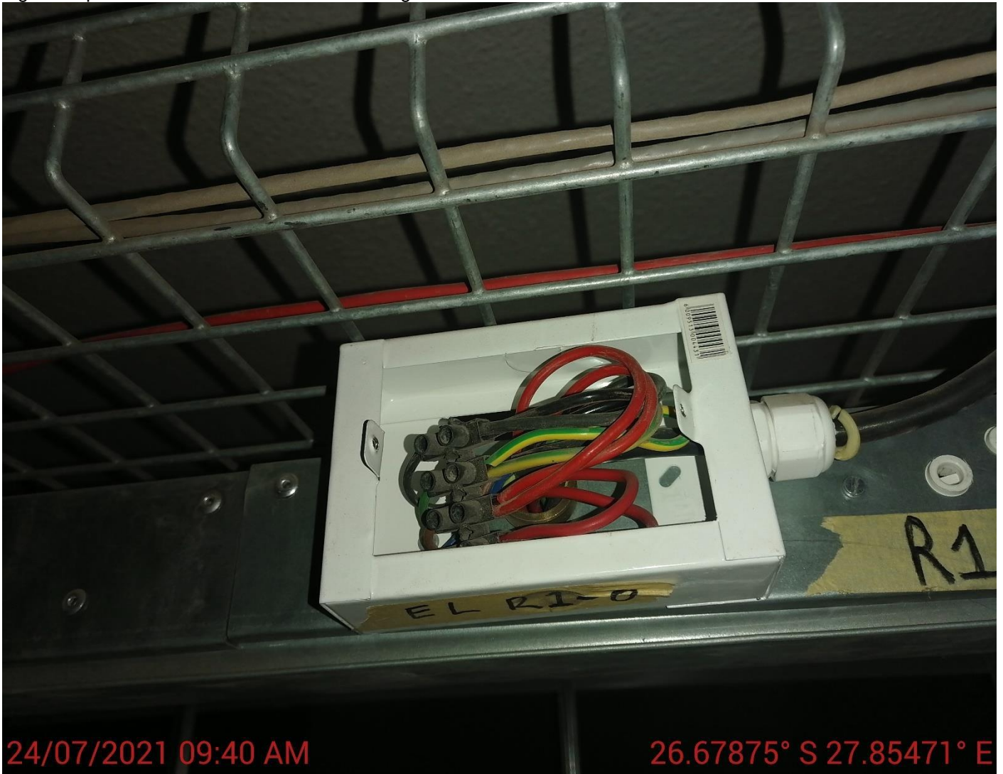
Fig 23 - Open Junction box – Tea Kitchen ceiling Void
