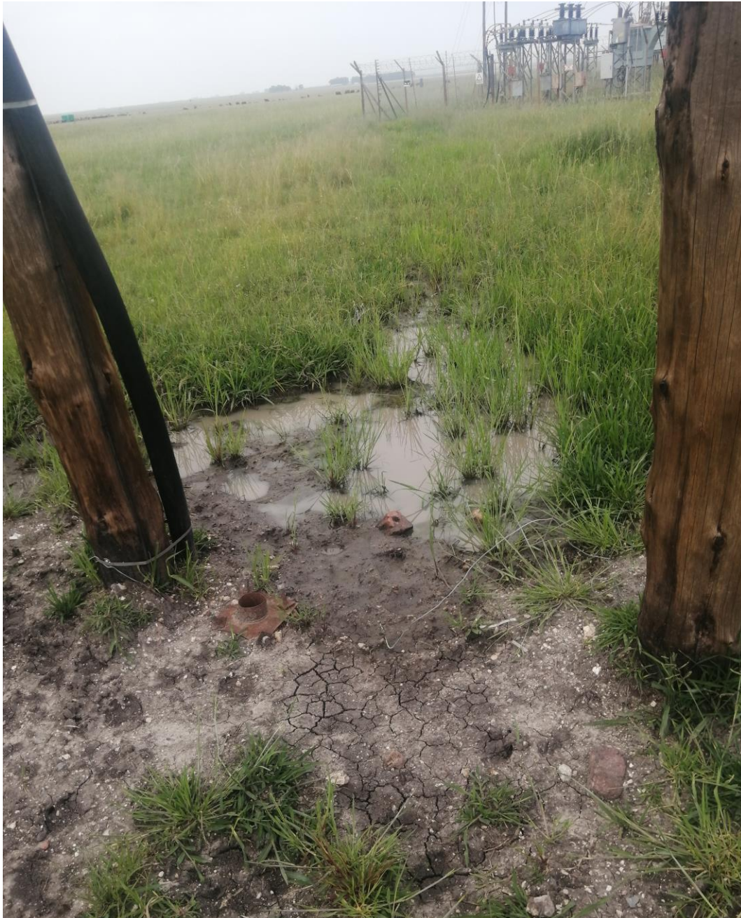
FIGURE 4: WATER DAMMING AT MV POLE CODE 2 OUTSIDE SUBSTATION
