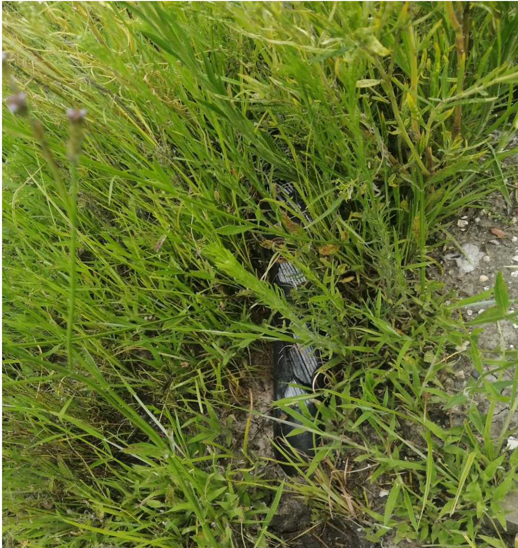
FIGURE 8: EXPOSED CABLE AT POLE NUMBER COWO 1
