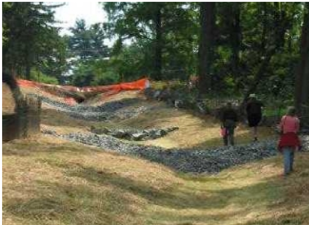
Figure 10: Rocks enclosed in wire walls (check dams)
