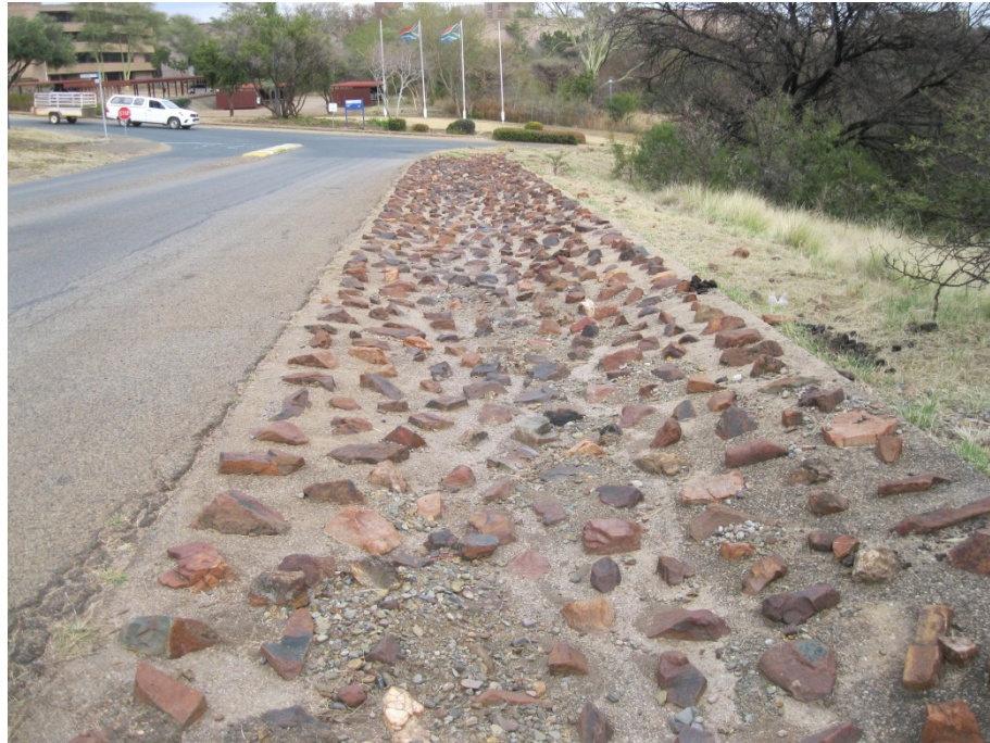
Figure 11: Rocks imbedded in concrete (preferable method)
