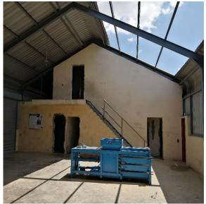
PHOTO 31: Stolen roof sheets and broken doors
