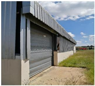
PHOTO 32: loose corners and side cladding
