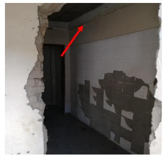
PHOTO 34: Damaged Wall tiles and ceiling
