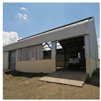
PHOTO 30: The main building with missing roofing and side cladding
