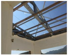
PHOTO 3:Light structural steel for the guard house
