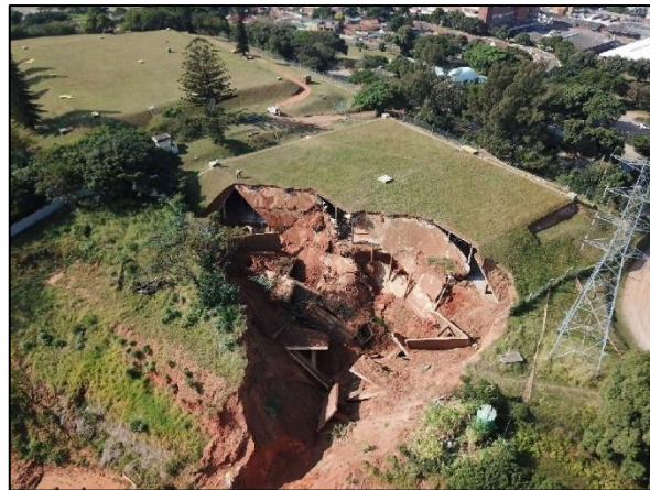
Plates 5 to 7: Remnants of the natural dune on the west of Reservoir 2 will yield borrow material for the new fill embankment
