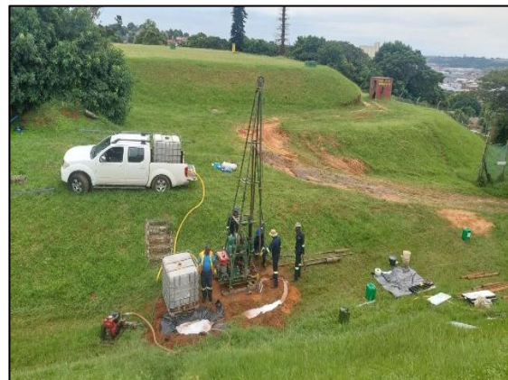
Plates 1 & 2: Boreholes BH1 and BH2 drilled along the southwestern and northwestern sides, respectively, of Reservoir 2
