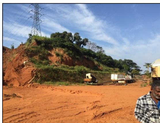
Plates 8 to 10: Pylon within 7m of the edge of the slipped surface
