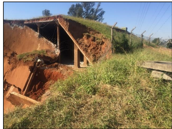
Plates 3 & 4: Damaged section of the reservoir near the southern corner, showing the platform abruptly truncated by the breach and the inside of the concrete chamber exposed.
