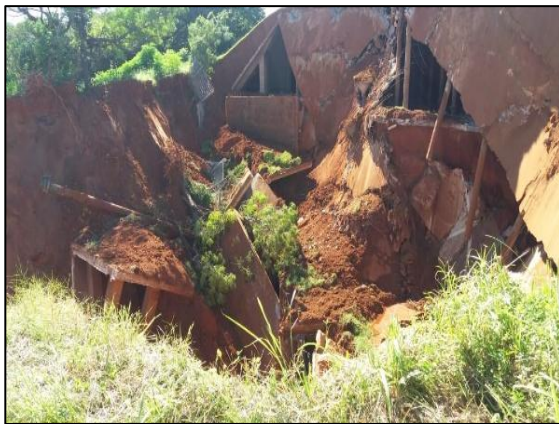
Plates 3 & 4: Damaged section of the reservoir near the southern corner, showing the platform abruptly truncated by the breach and the inside of the concrete chamber exposed.
