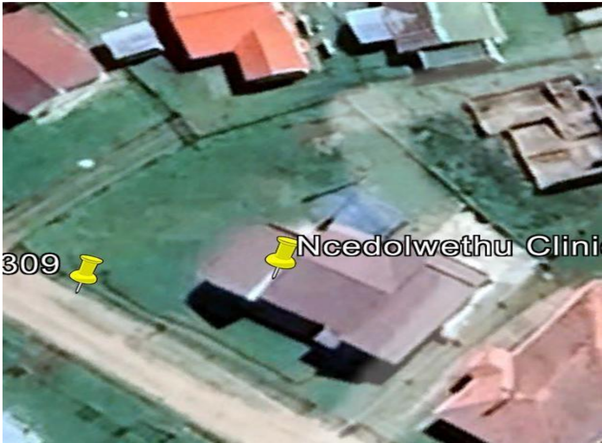
NCEDOLWETHU CLINIC AERIAL VIEW (SOURCE GOOGLE EARTH)
