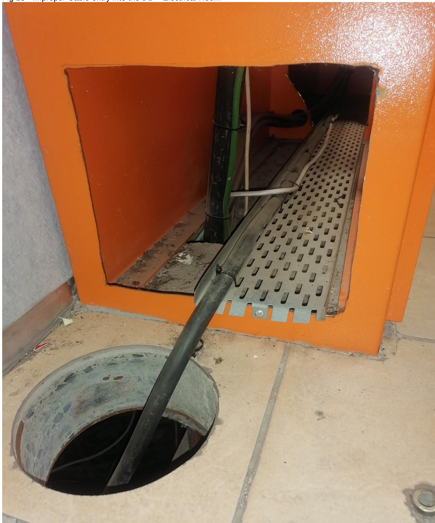
Fig 18 - Improper Cable entry into the DB – Electrical Room
