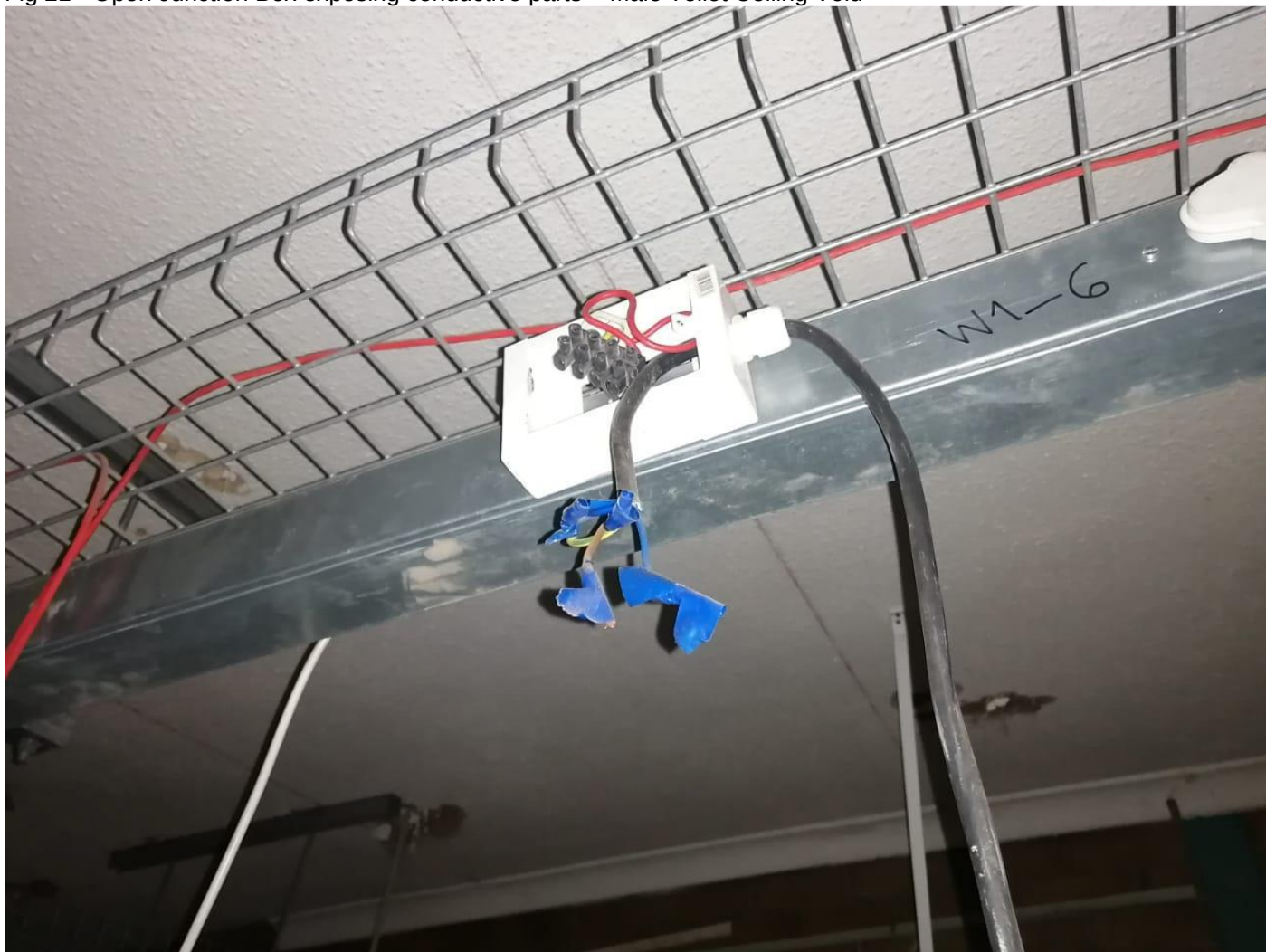
Fig 21 - Open Junction Box exposing conductive parts – Male Toilet Ceiling Void
