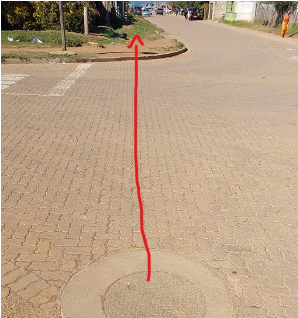
Figure 4: Manhole at starting point.
