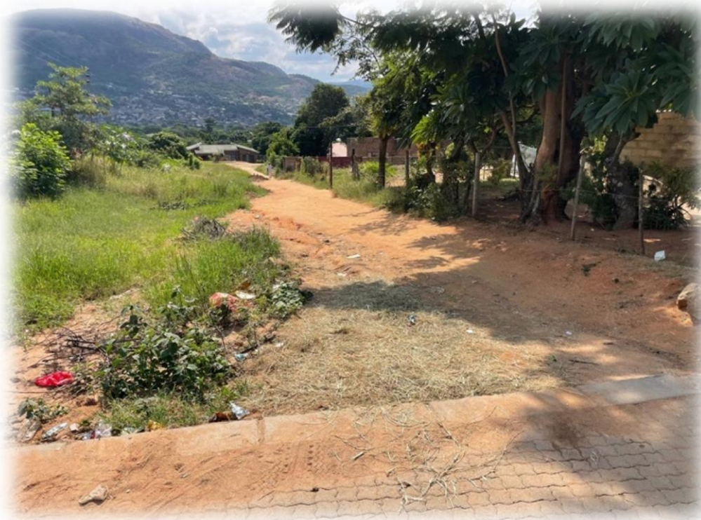
Figure 4 – Eroded road due to runoff
