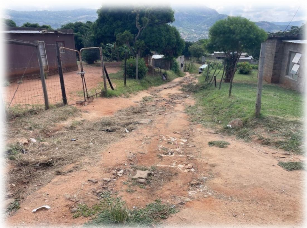
Figure 2 – Narrow road width, boundary fences to be relocated.
