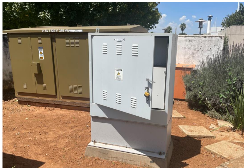
Figure 4: Matumi Building 500kVA LPU Meter Kiosk
