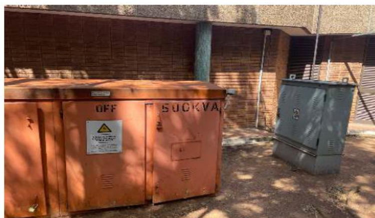
Figure 3: Security Office Mini-Substation 11kV Meter Kiosk
