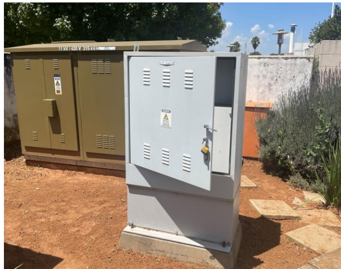
Figure 2: National Control LPU Meter Kiosk
